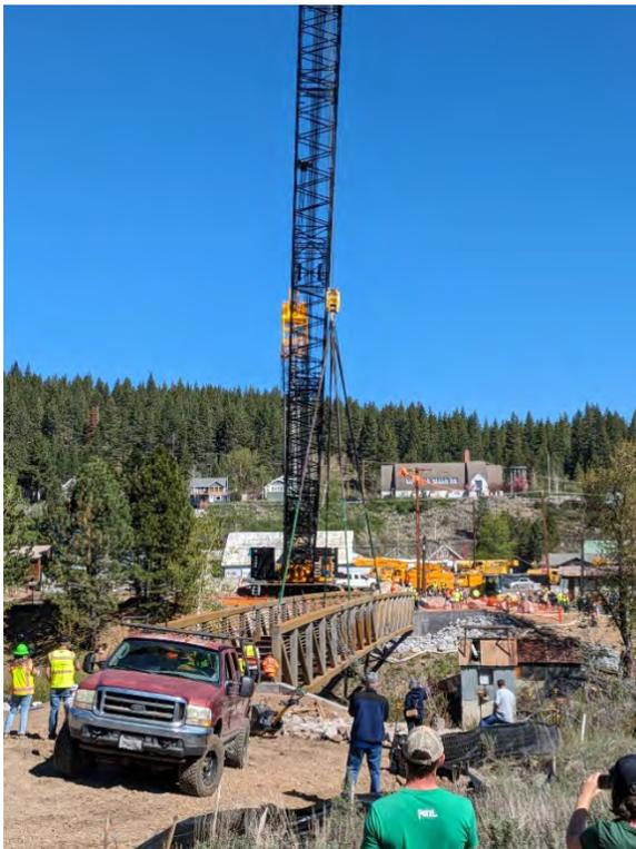
*Figure 5: New Pedestrian Bridge installation for Legacy Trail*
